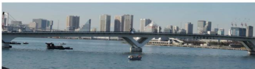
Fig. 1.19 The Toyosu Bridge in Tokyo, Japan. (Photo by Zheng.)
