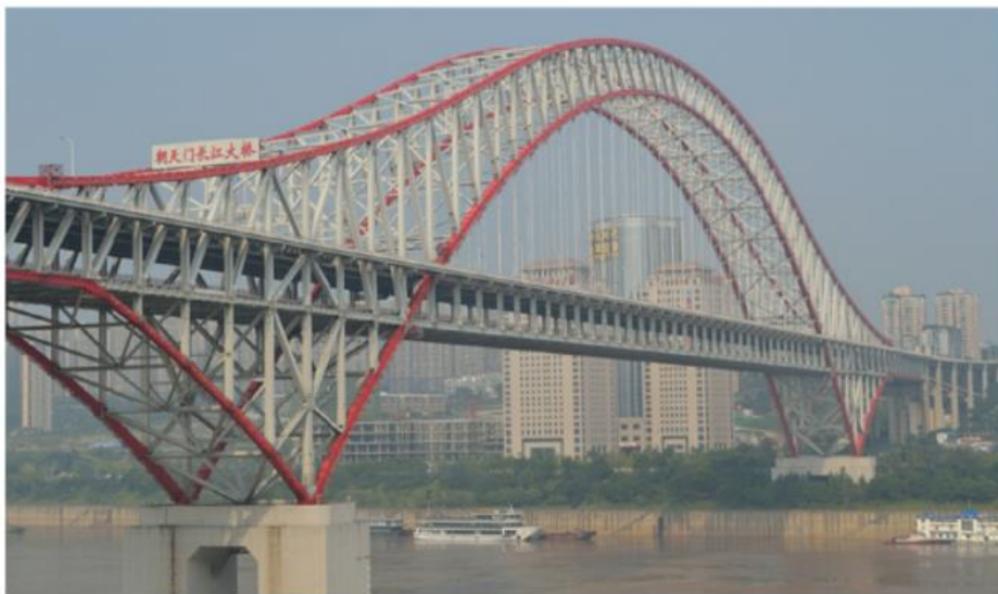
Fig. 1.22 The Chaotianmen Bridge, Chongqing, China. (Photo by Yan.)
