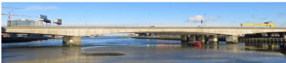
Fig. 1.16 Lagan bridge (concrete continuous girder bridge), Belfast.
