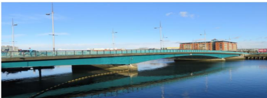
Fig. 1.17 Queen Elizabeth II Bridge (steel continuous girder bridge), Belfast.
