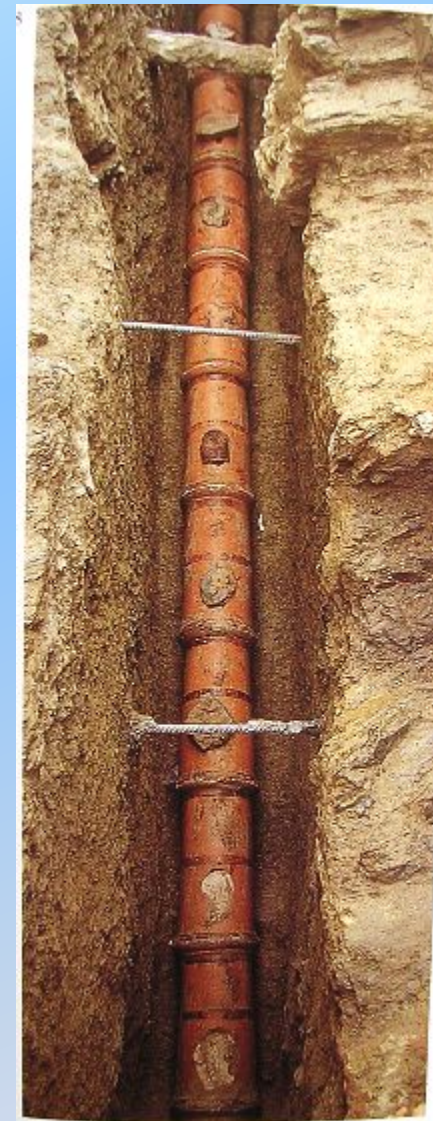
8. SYNTAGMA Station. Part of the "Pisistratan" pipeline.
