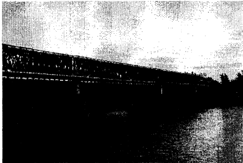
Old Bridge (Truss bridge)
