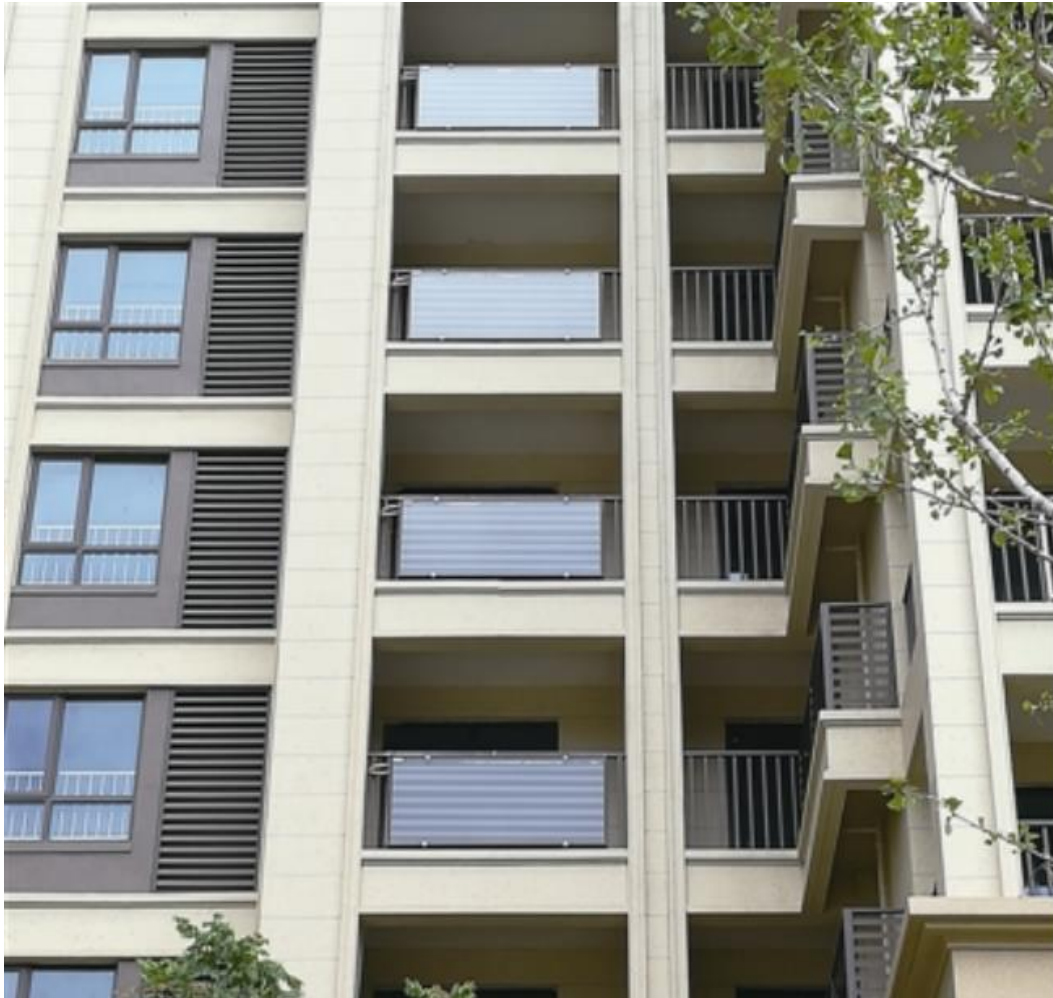
Figure 2 – Curved surface heat absorption solar water heater
