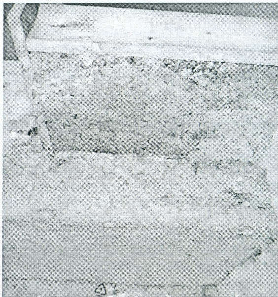
Fig. 1. Samples of lime-silicate heat insulating fiber-reinforced concrete with organic fiber fillers of vegetable origin
