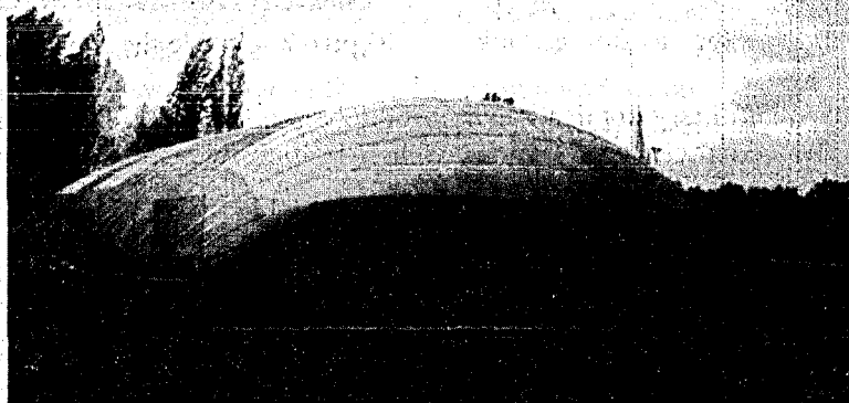
Figure 5 – The tennis hall in Chorzów (Poland)
