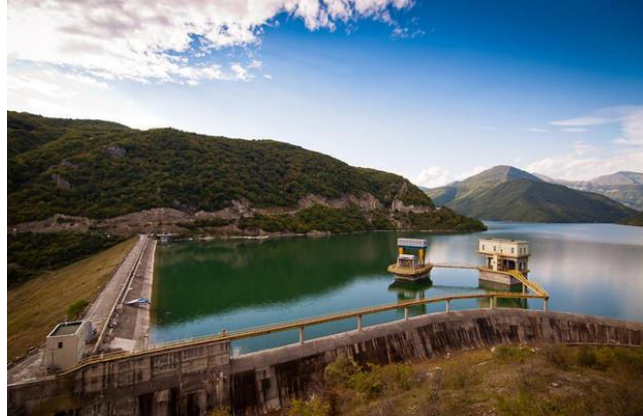
Figure 6 – The general view of the Zhinvali Earth Dam
